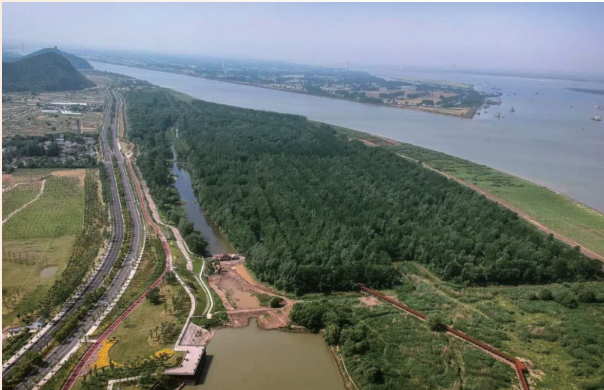
Riverside Wetland Park renovation project supported by Anhui Branch
