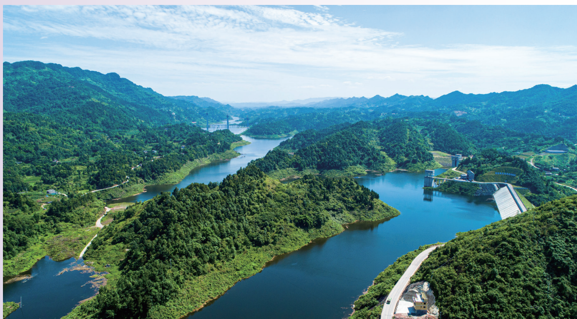
Guanjingkou water conservancy project supported by Chongqing branch
